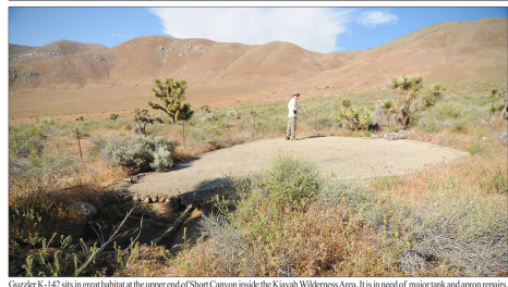
Guzzler K-142 sits in great habitat at the upper end of Short Canyon inside the Kavah Wilderness Area. It is in need of major tank and apron repairs.
